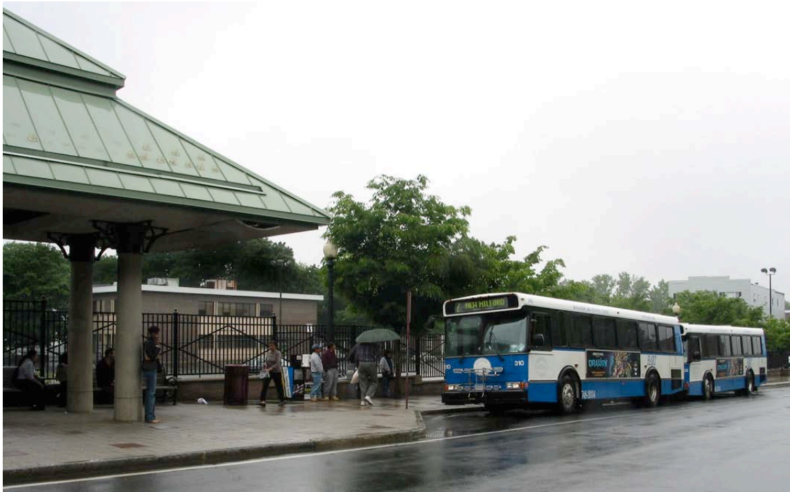
Front bays at HART Kennedy Avenue Pulse Point, looking towards Main Street, Danbury.
