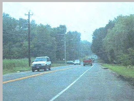
Route 35 between Copps Hill Road and Route 7 with striped shoulders approximately 6 feet wide
